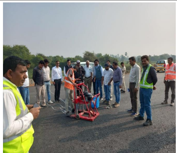
Core Cutting of DBM Top at ch. 356+800 during Site Visit
