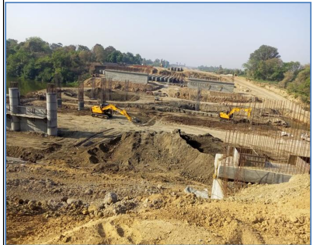
Work in Progress at MJB @ 358+050
