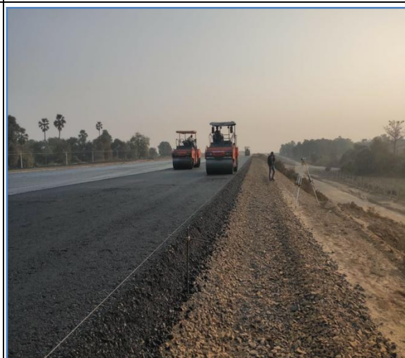
DBM Top Laying at ch. 357+400 to 357+800
