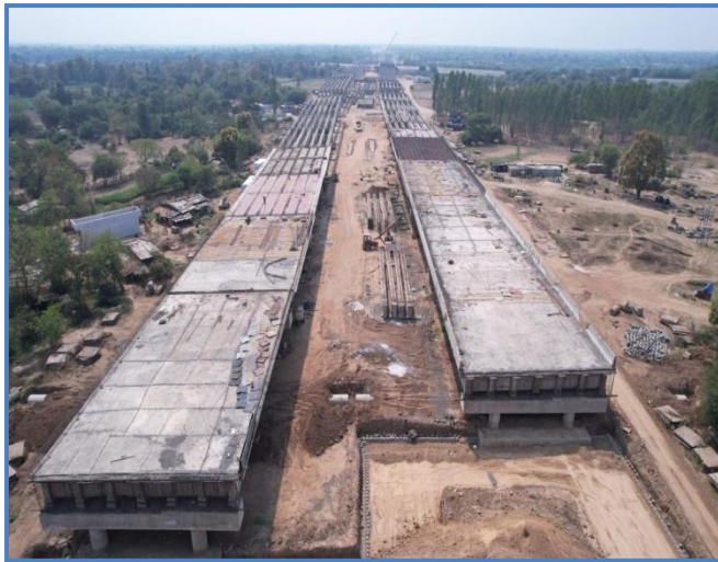
Casting of Deck Slab A1 side @ 352+281
