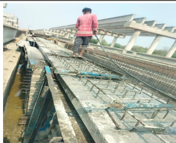
Girder Curing at casting yard
