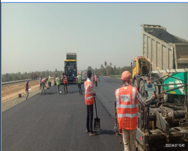
DBM Top Laying at chainage – 357+400 to 357+850
