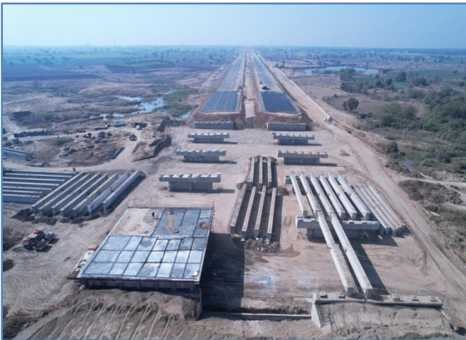
Casting of Deck Slab @ 359+936
