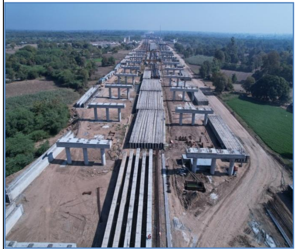
Casting of Girder A2 side @ 352+281
